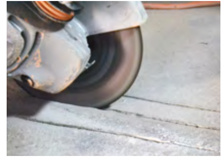
Creation of traces on reinforced concrete.
